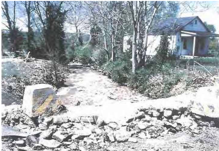
Destruction of Street and Blockage of Culvert with Debris and Sediment on Pedlar Gap Run from April 1992 Flood
