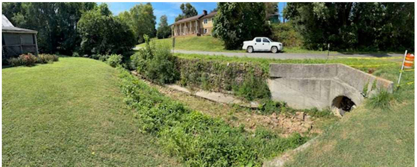
Vegetated Gabion Wall at Woodland Ave Culvert (Constructed Circa 1977)
