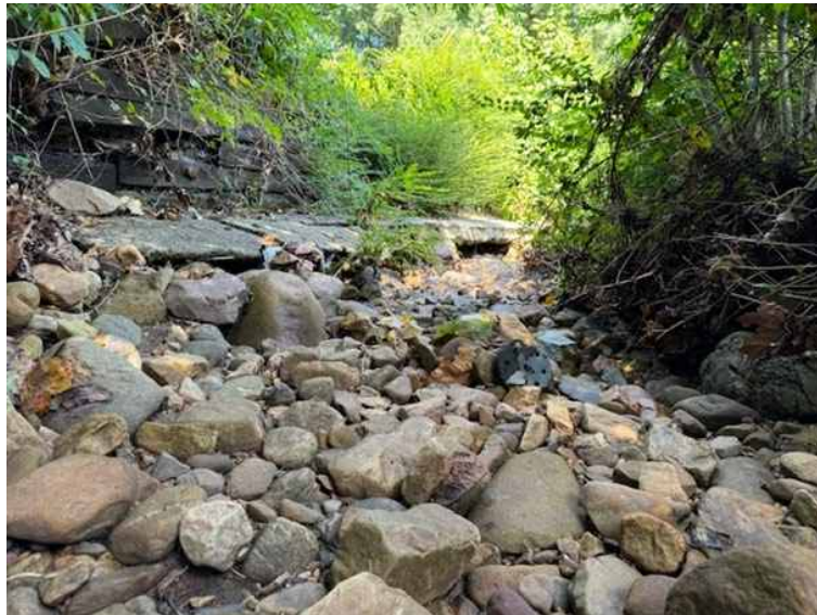
Wooden Crib Wall at Left, High Flow Concrete Overbank, and Low Flow Natural Channel with Cobbles
