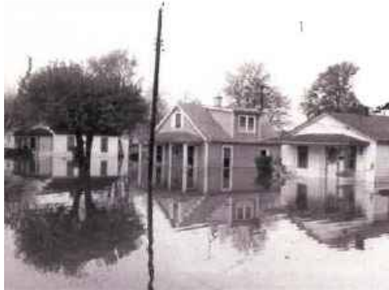
Flooding at Forest Avenue 1992
