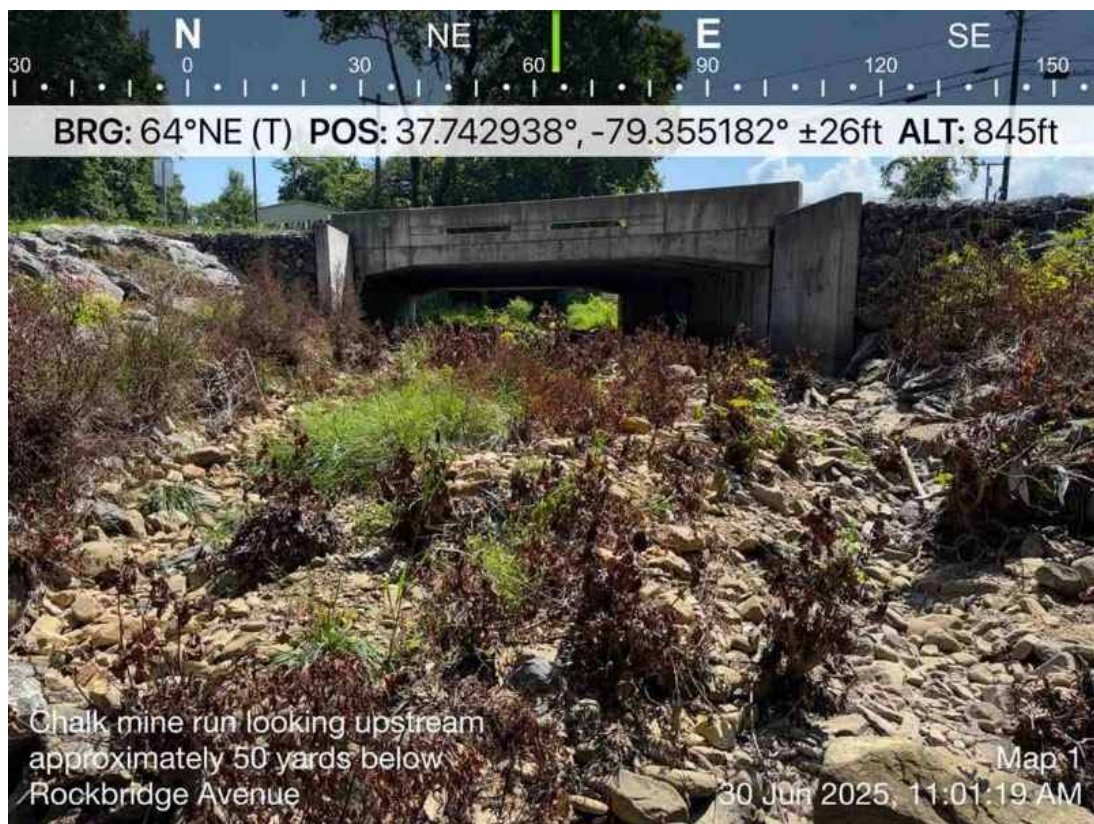
Rockbridge Avenue Bridge Circa 2025
