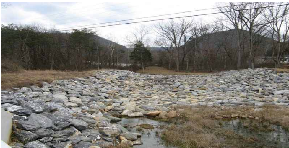
Debris Basin on Chalkmine Run shortly after construction
