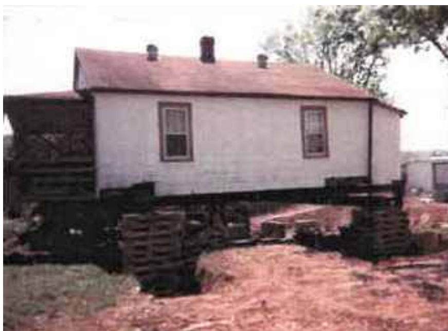
Home Being Elevated
