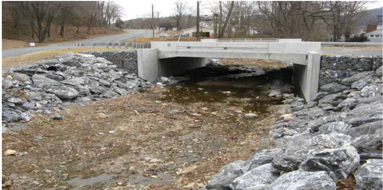
Rockbridge Avenue Bridge Circa 2010
