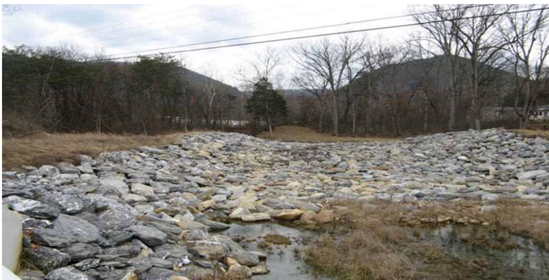
Chalkmine Run Debris Basin Circa 2010
