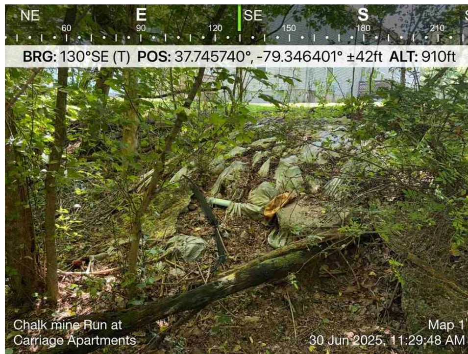
Rip-Rap Covered by a Tarp Reinforcing the Embankment Behind Carriage House Apartments
