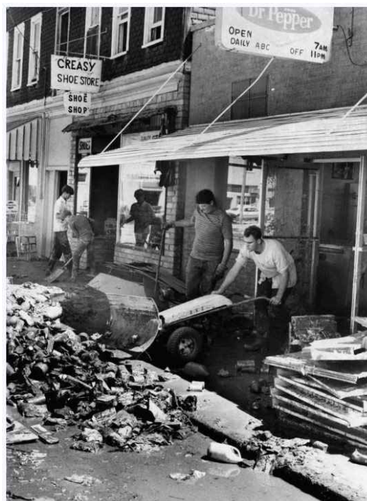
Downtown Buena Vista Cleanup following Hurricane Camille. Credit: Gene Carrow from the Richmond Times-Dispatch
