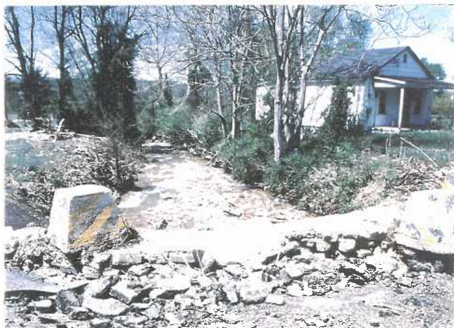
Destruction of street and blockage of street culvert with debris and sediment on Pedlar Gap Run from April 1992 flood.
