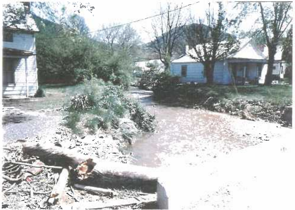
Debris and sediment blocking street culvert near confluence of Noels and Indian Gap Runs after April 1992 flooding.
