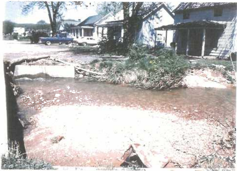
Sediment and debris blocking street culvert on Noels Run after April 1992 flooding.
