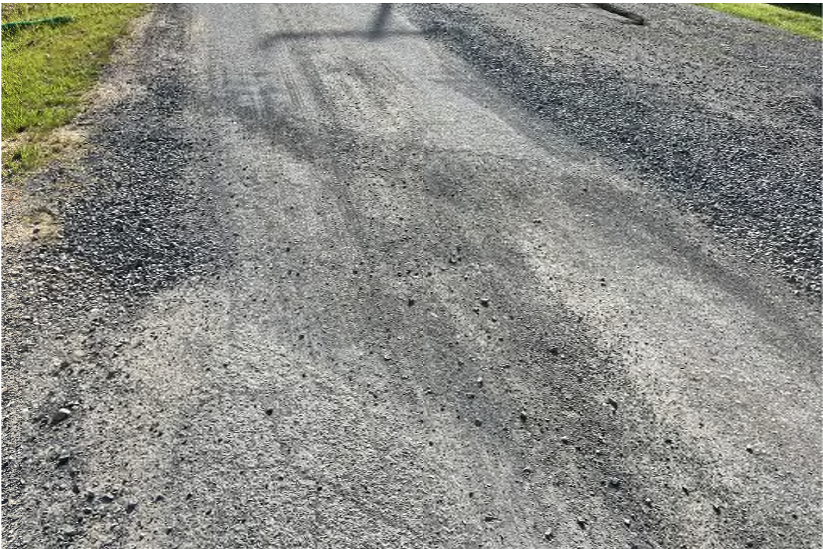
32nd St pavement cut for drain pipe
