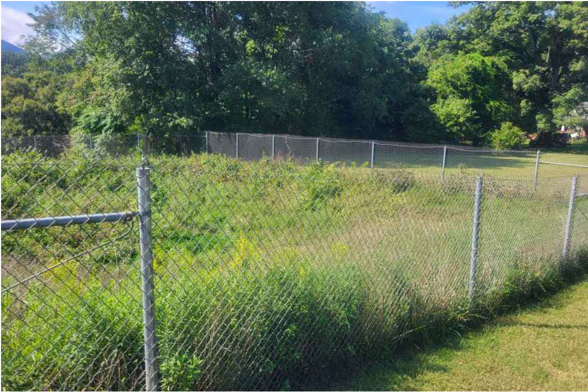
LOOKING FROM CATALPA AVE WEST SHOWING STORM WATER POND
