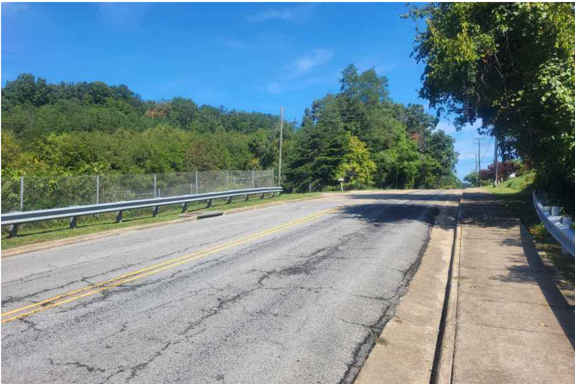
LOOKING NORTH ON CATALPA AT LOCATION OF ENTRANCE
