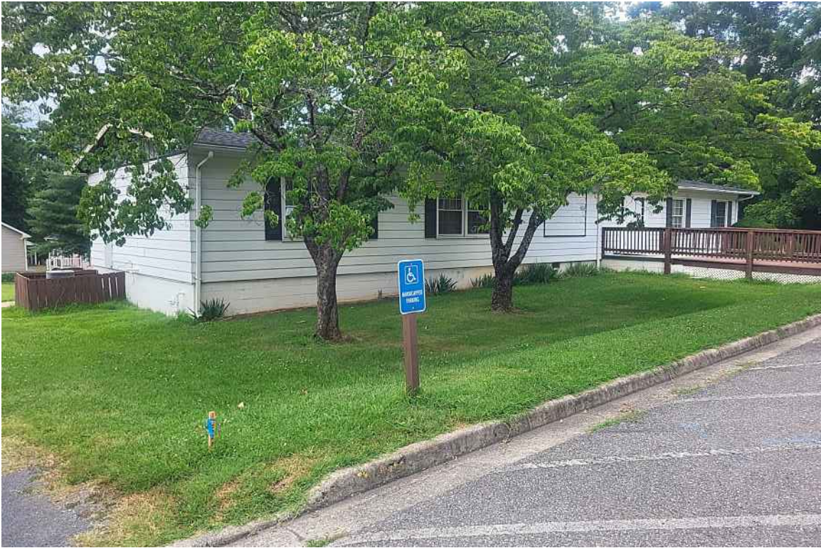
115 Ridge Ave, to be demolished
