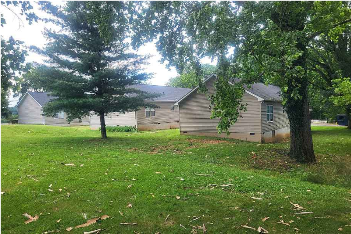
Modular dorms to be demolished, looking from behind 115 Ridge Ave west; new building will be straight ahead
