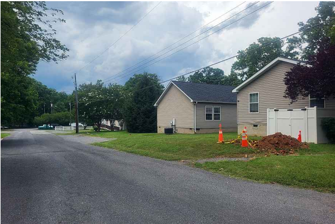
Modular dorms, looking northwest from 27th St near Magnolia Ave
