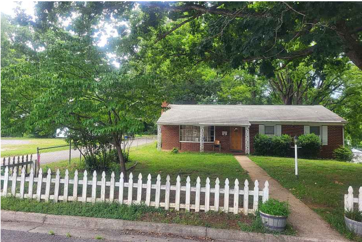
212 W 27th St, to be demolished, looking west
