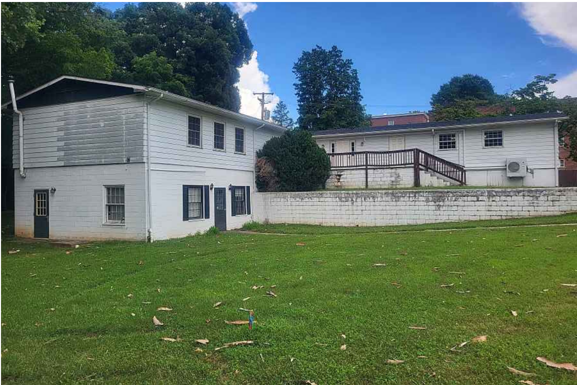
115 Ridge Ave rear, to be demolished
