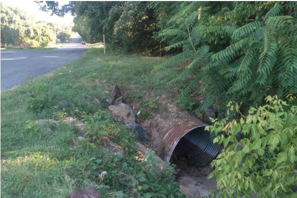
CULVERT OUTFALL - PEDLAR GAP RUN ON WEST SIDE OF WOODLAND AVE
