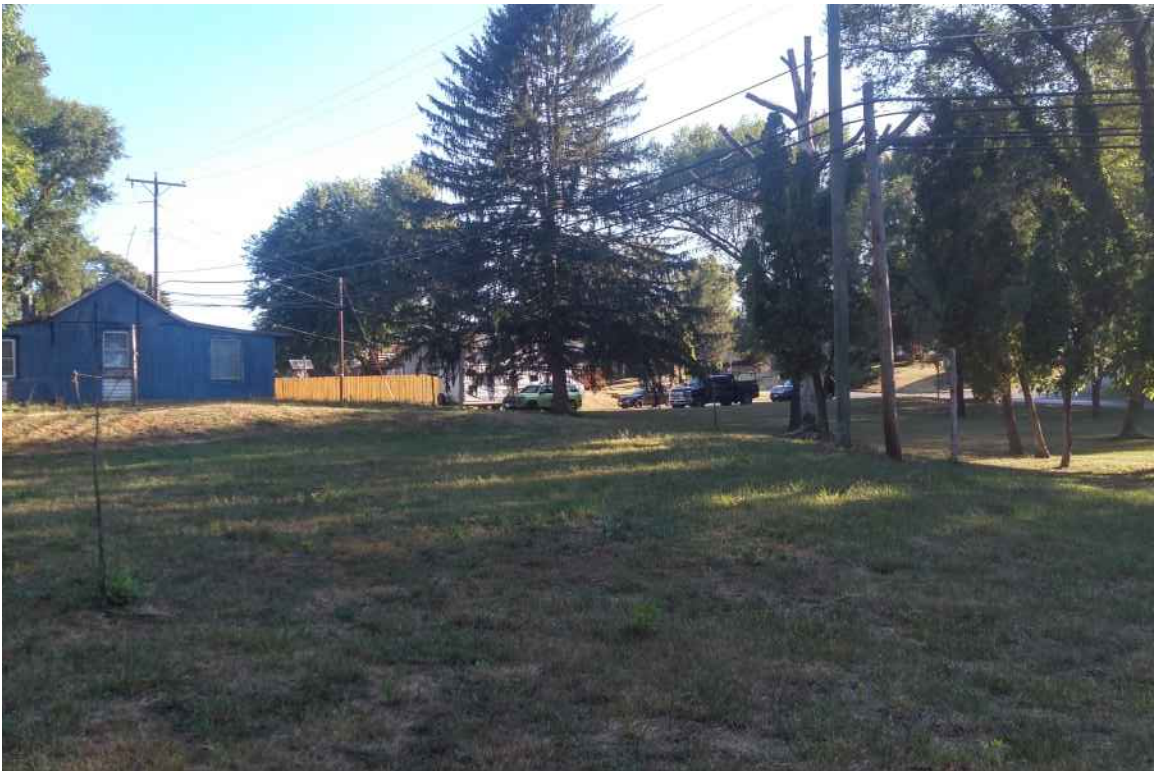
ON SITE LOOKING SOUTH TOWARD 6TH ST. HOUSE AT LEFT TO BE DEMOLISHED
