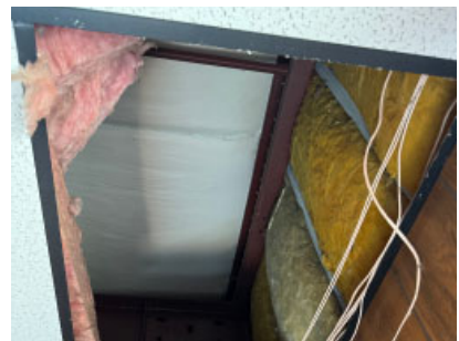
Section A: Typical roof insulation.
