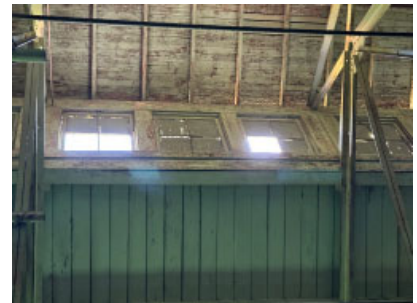
Section D: Monitor window along roof ridge.
