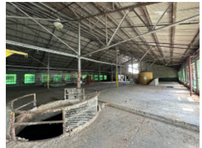
Section I, Second Floor: Roof structure.
