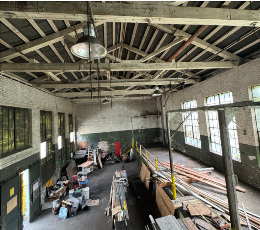
Section B: View from mezzanine in Room 2.
