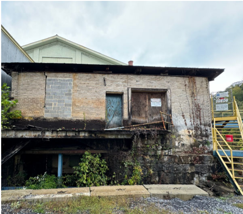
Section M: West wall.
