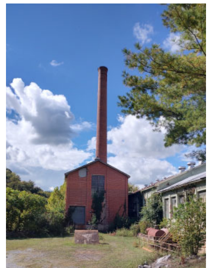
Section G: View from east, brick chimney visible behind the structure.
