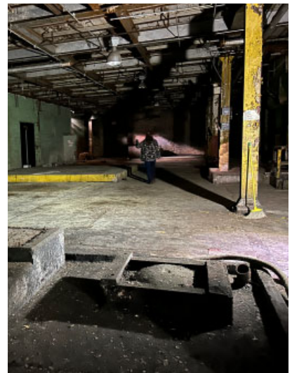
Section L: First floor columns and concrete curbs.
