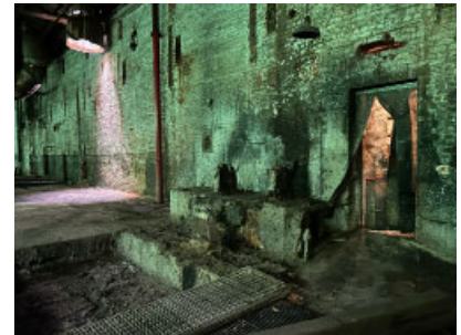
Section H: South wall at connection to Section I.
