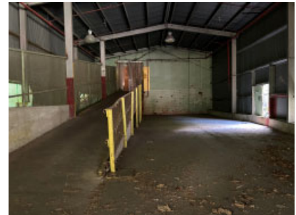
Section N: Ramp to Section L.
