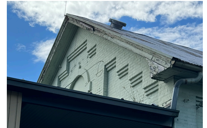
Gable end of Section D showing decorative brickwork.
