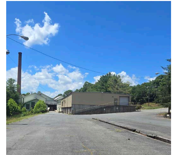
East end of building, with Route 60 access to the right.
