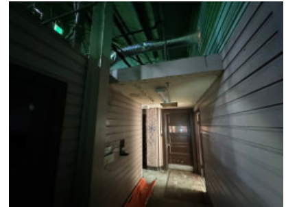
Section D: Office space hallway with original wood siding and doors.
