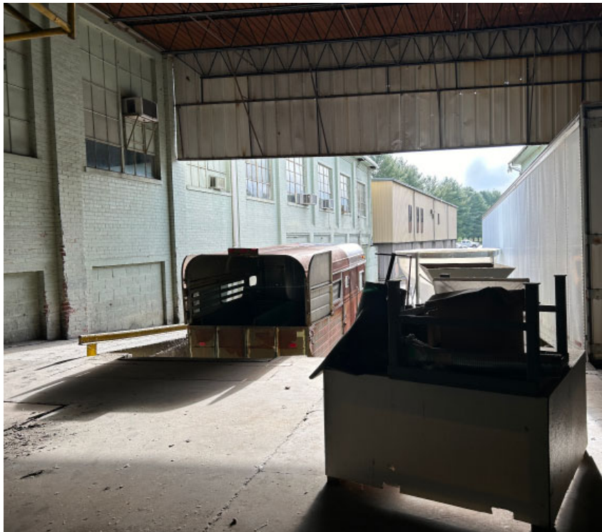
Section C: Platform lift that accesses Section D.
