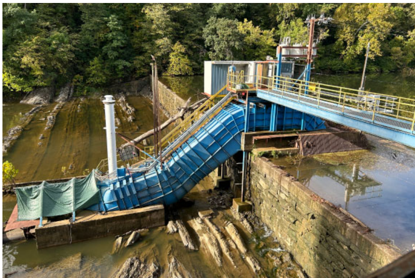
Hydroelectric dam at the Maury River. Operation of this dam is independent of the Bontex site.
