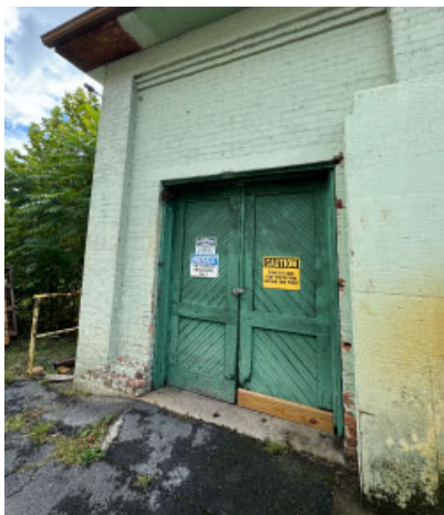
Section B: Original exterior freight door at east end, Room 1 access.
