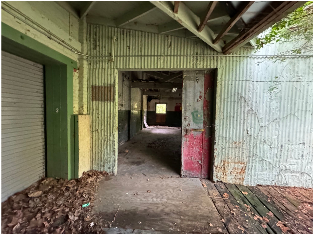
Section K: North wall and partial interior view.
