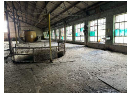
Section L: South wall.
