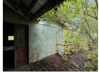
Section K: Northwest corner and wood catwalk.
