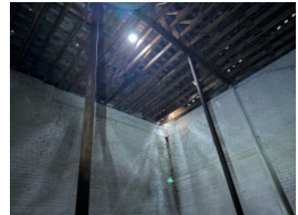
Section I: South room wood roof framing and hole.
