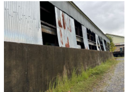
Section N: Typical exterior wall condition, continues along Section O.
