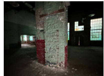
Section E/F: West half brick pier.
