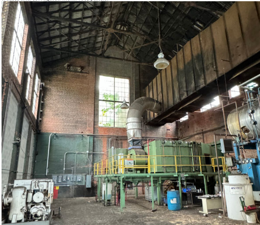
Section G: View looking west.
