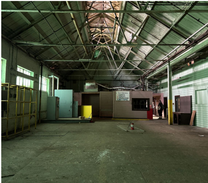
Section D: Looking east towards offices.
