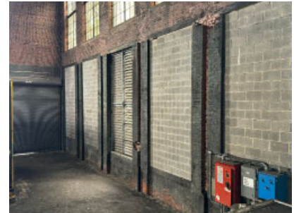
Section G: CMU infilled window openings.
