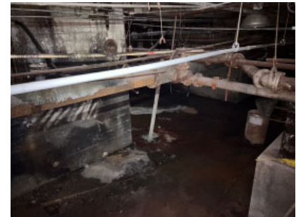
Section I: Basement condition.
