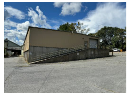
East end of mill building. Site grade slopes gradually uphill towards Rt. 60.
