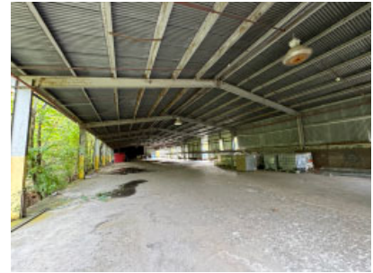
Section O. looking east towards Section N.
