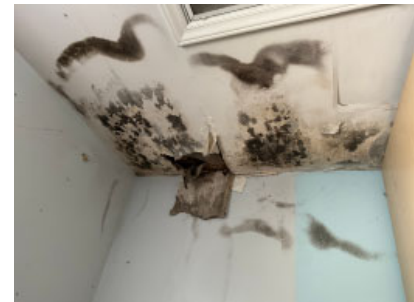
Section D Laboratory: Black mold.
