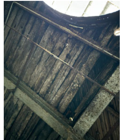
Section I: Underside of second floor structure.
