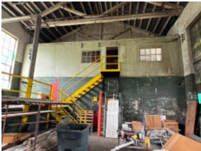
Section B: View of mezzanine level office area.
