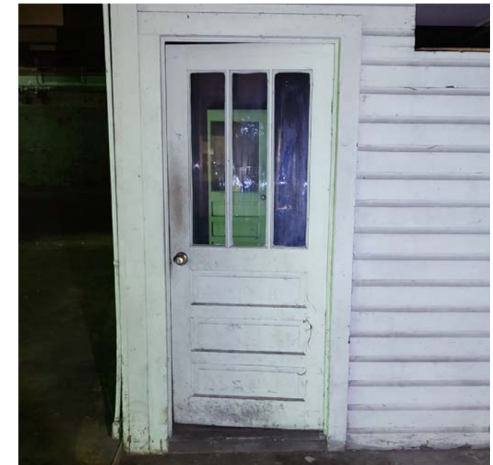
Original office door with wood siding, Section E/F.
