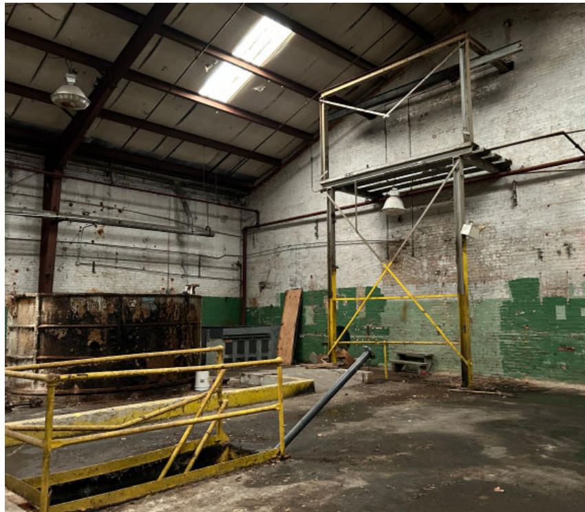
Section I: Northeast corner.
