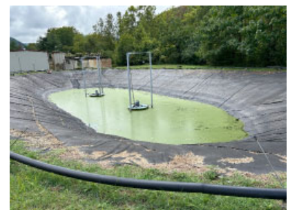
Water treatment reservoir.
