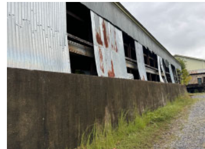
Section O: North side metal siding.
