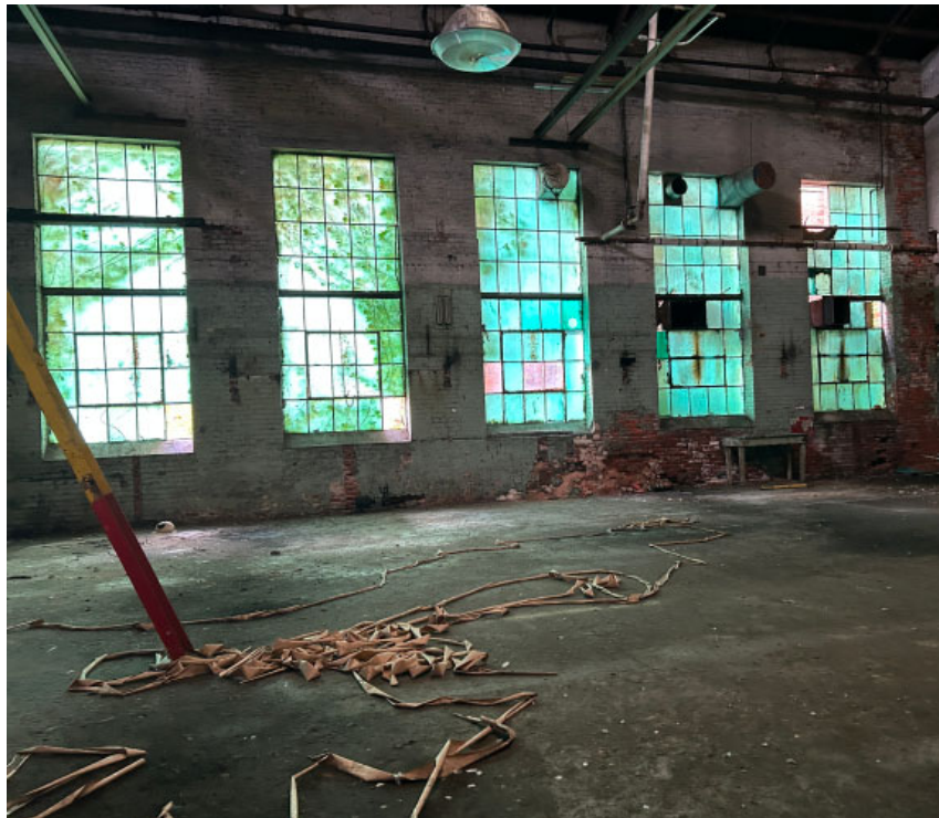
Section E/F: South wall, with room division on the right side.
