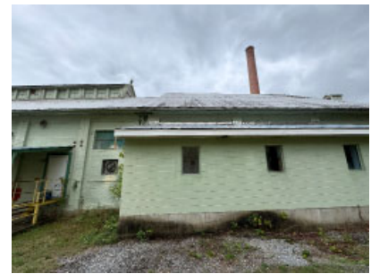
Section D: Typical roof condition observed on site.
