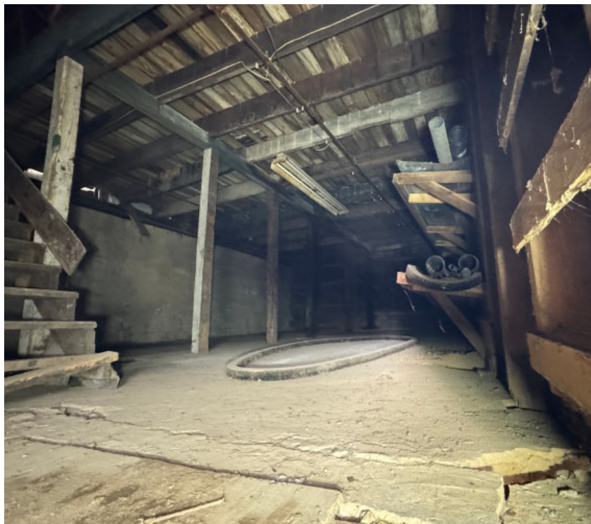
Building X: Interior condition.
