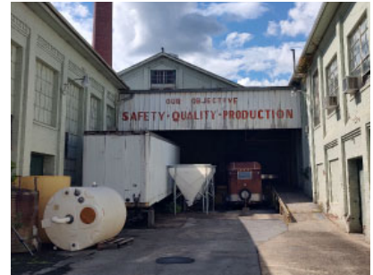
Section C: View from service drive, looking at loading area.
