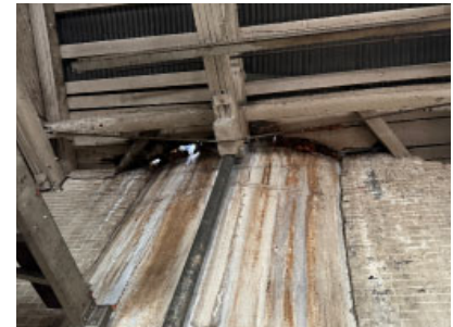
Section B: Tank integrated into wall structure in Room 2.
