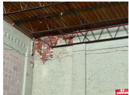
Section C: Southwest corner roof condition.
