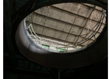
Section L: Round floor opening, looking toward roof from first floor.
