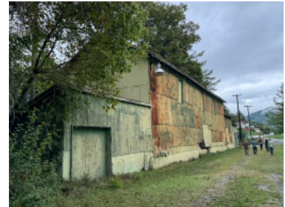
Building X: View of south wall.
