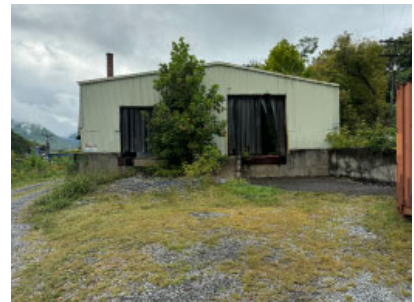
Section O: West End Loading Docks
