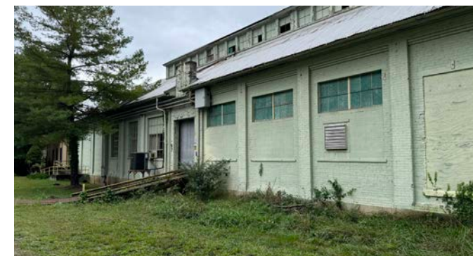
North side of Section D.
