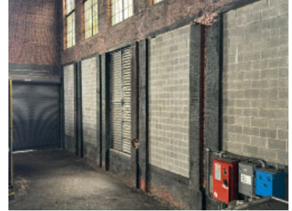
Section G: CMU block infill at original window openings.
