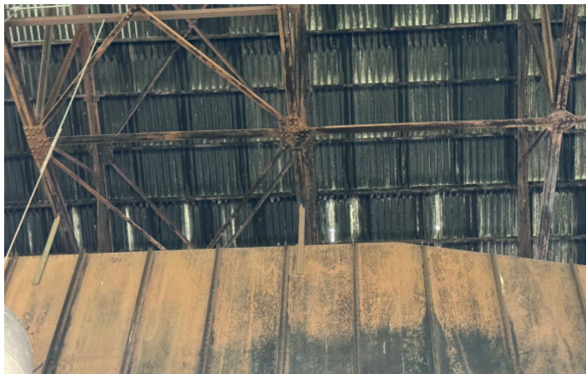
Section G: Roof and framing condition.
