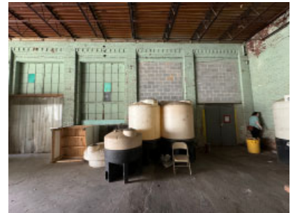
Section C: South wall, which is the exterior of Section B.
