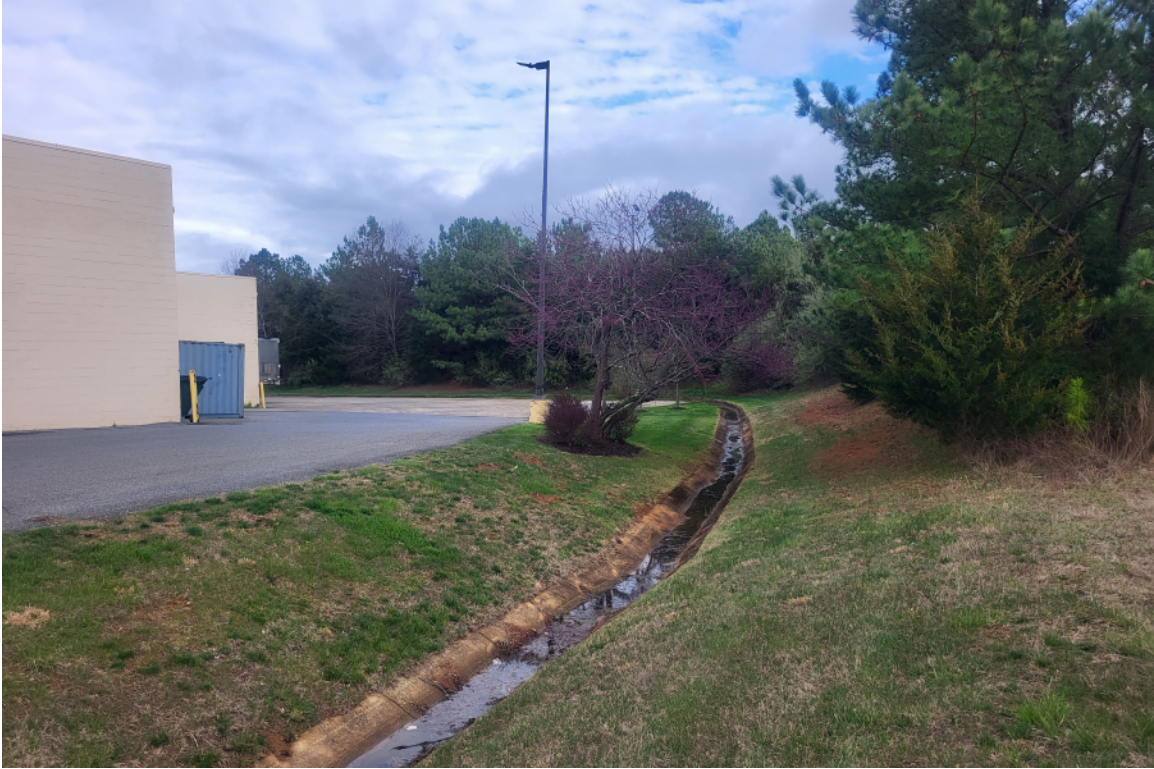
AT WESTERN ENTRANCE LOOKING SOUTH AT TREES SCREENING PROPERTY FROM FOOD LION
